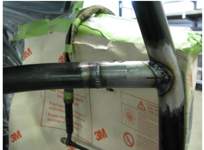
Figure 13 – Finished Cross Brace
