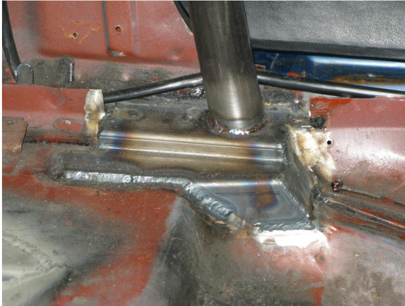
Figure 2 – Rocker Doubler Installed
