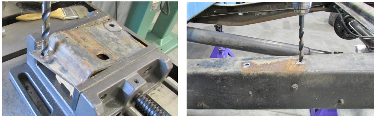
Figure 2 - Drill Out Brackets & Frame Rails
