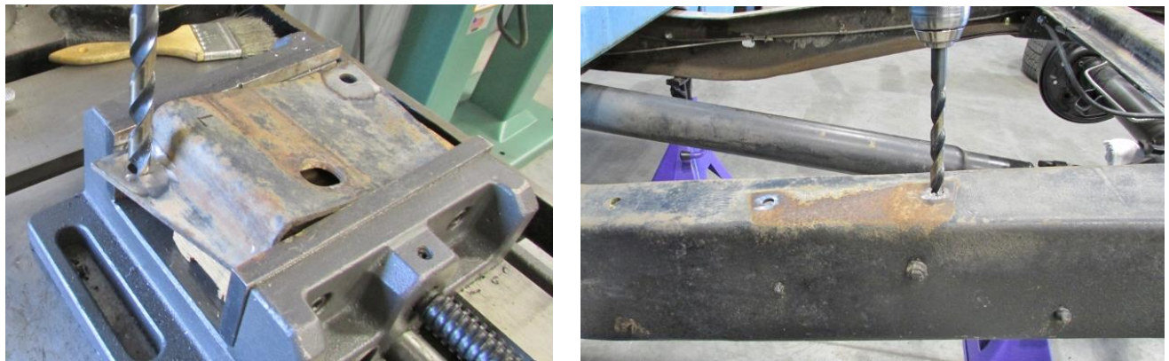
Figure 2 - Drill Out Brackets & Frame Rails
