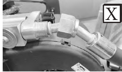
Improperly Seated O-ring Land
