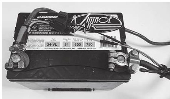
Completed Installation Shown
