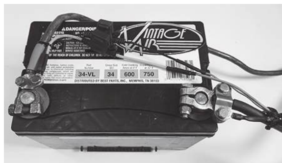
Completed Installation Shown
