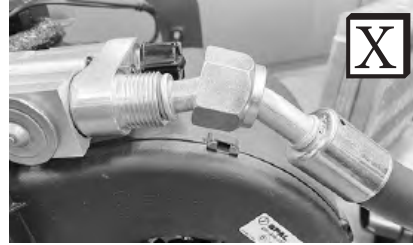
Improperly Seated O-ring Land
