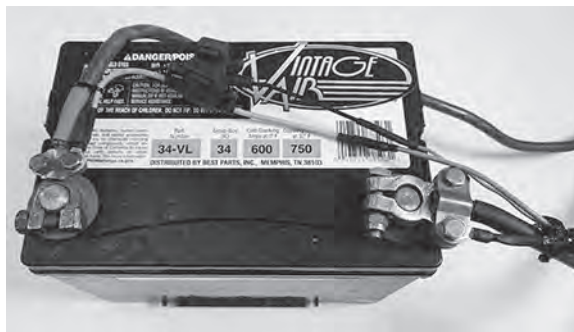
Completed Installation Shown
