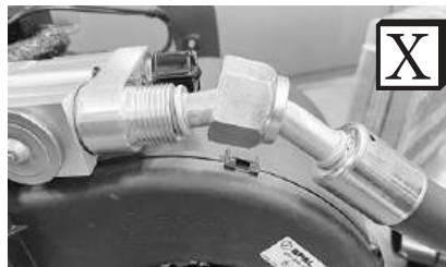
Improperly Seated O-ring Land
