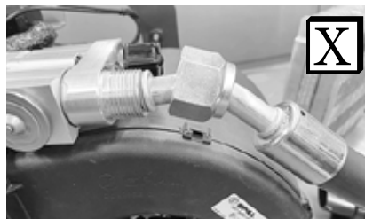
Improperly Seated O-ring Land
