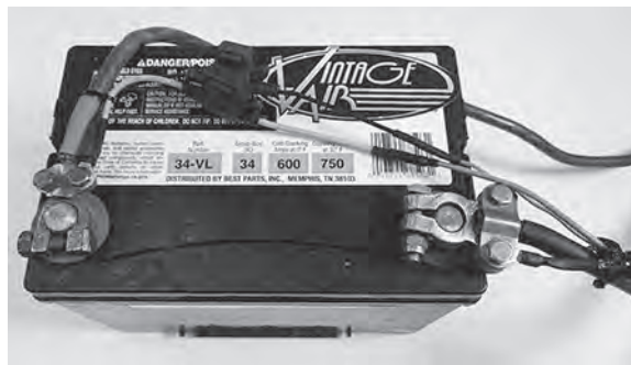
Completed Installation Shown
