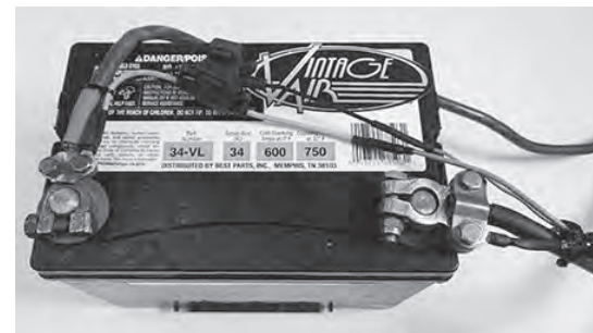
Completed Installation Shown
