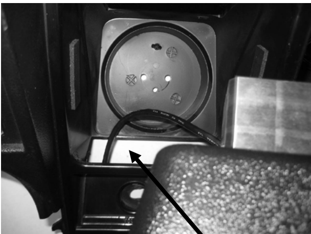
Cable routed through indicator light opening
